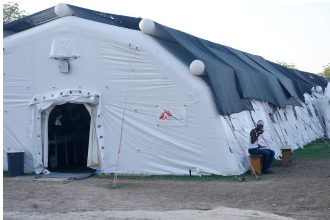
Figure 2-2. An inflatable structure used by Mediciens Sans Frontieres for a hospital after an earthquake in Haiti. Image credit www.doctorswithoutborders.org
